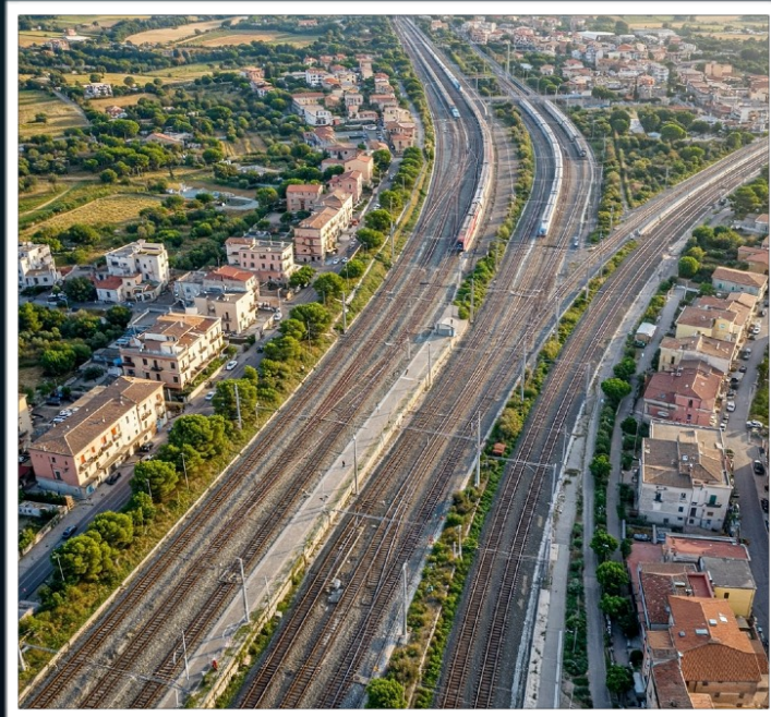
Messina Tramway – New tramway construction project
