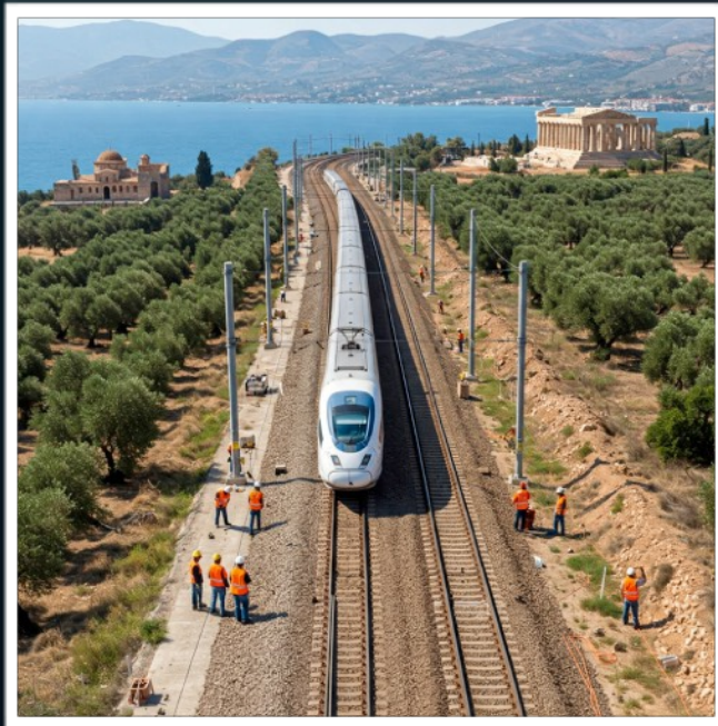
Railway project in Greece
